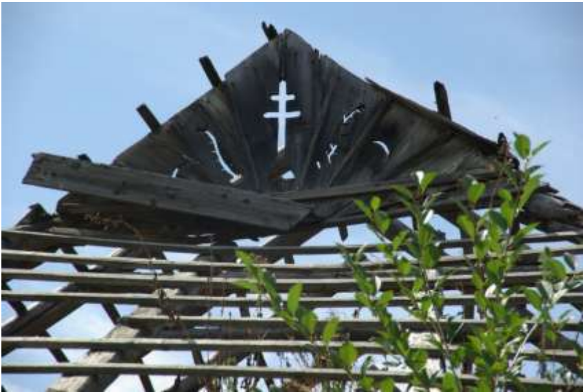
Figure 4. Open street view, only the pediment remains from the roof, the tree grew out of the wall
